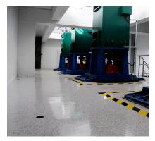
Tnemec's Series 224 Deco-Fleck, a flake-filled polyamine epoxy floor topping, was the solution to the flooring needs at the Pudong Waigaoqiao No.3 Pump Station.
