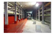
The underground trenches at the Baosteel manufacturing facilty received a finish coat of Series 282 Tneme-Glaze to protect the concrete from leaks and overflows of harsh chemicals.
