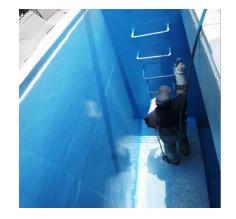
A waste acid and emissions collection process was developed by Baosteel with the intent of handling a myriad of waste products. Series 365 Tank Armor was used to protect the concrete in containment pools.
